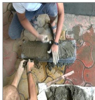
c. Application of Mortar
