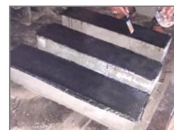
b. Layer of CFRP Sheet
