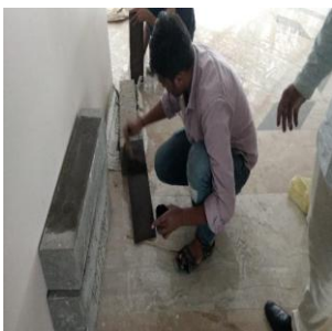
a. Application of Bonding Agent on the Surface.
