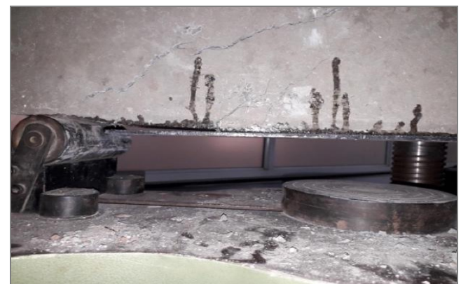
c. Beam with Steel Plate Bonding
