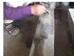
a. Application of Epoxy
