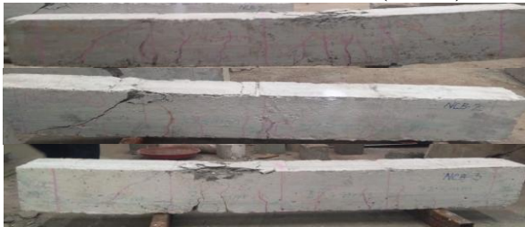
Fig. 14. Crack Pattern for Normal RC Beams (NRCB)
