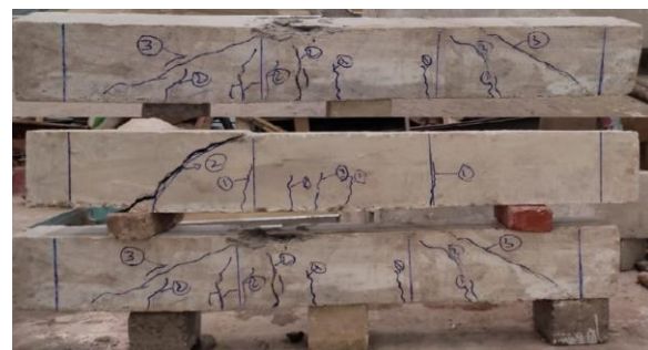
Fig. 16. Crack Pattern for DP+QDRC Beams.
