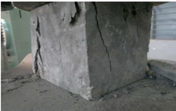
Fig B.2: Testing of Cube in UTM Machine
